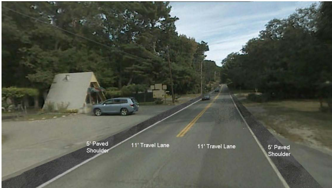
Figure 3 Example of 5' Paved Shoulders
