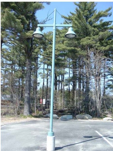
These light fixtures, recently installed at a local business, effectively light the parking lot with beams of light focused downward from shorter fixtures.
