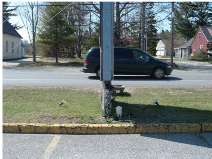
The spotlights used to light this sign are placed on the ground and shine upwards. Consequently, much of the light reflects or escapes into the sky.
