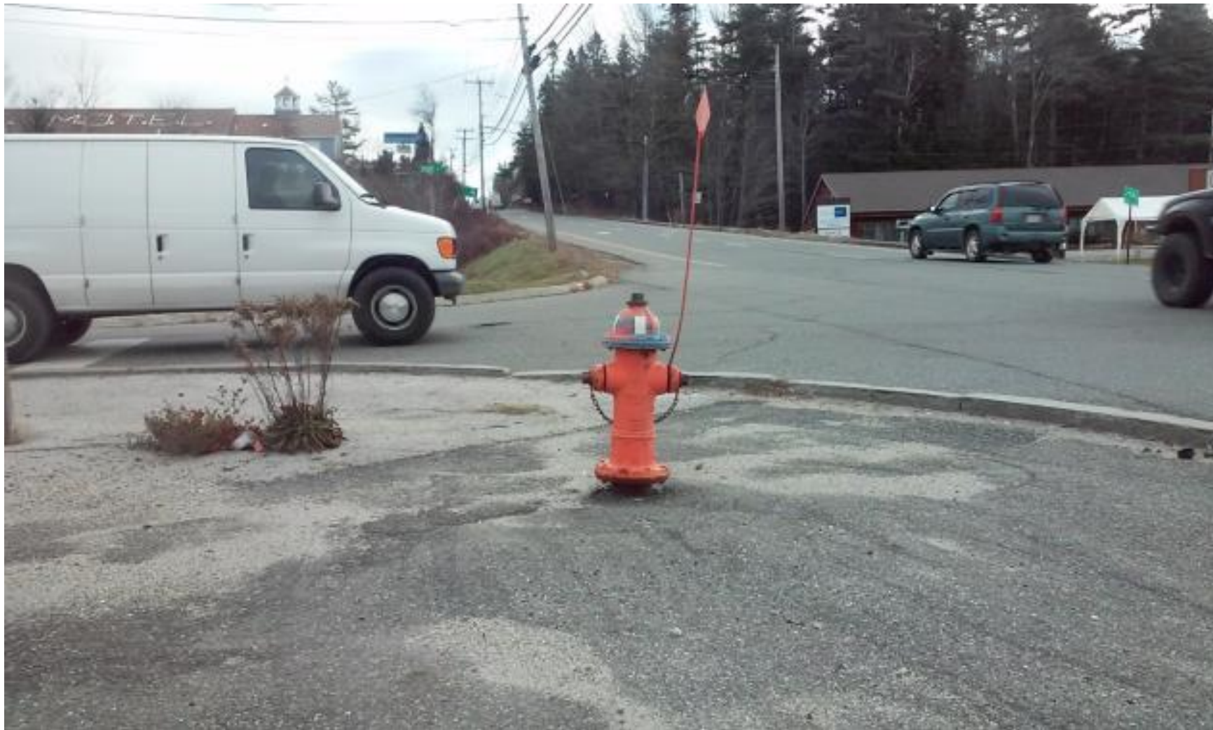
Photo C. Motorists on Short Street waiting to turn often pull close to High Street to enhance their view of oncoming traffic. Note the location of the painted stop line beneath the rear axle of the stopped vehicle in this photo.
